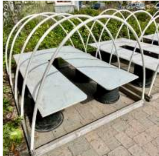
10' PVC pipes slip over the 60d nails.
